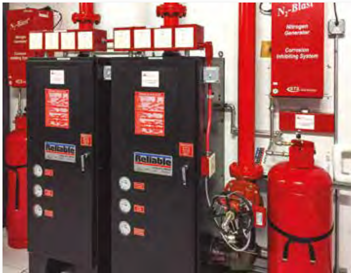
South-Tek N 2 -Blast® Nitrogen Generator fitted to a Reliable Model DDX PrePak Preaction System and Model DDX Preaction Valve.
