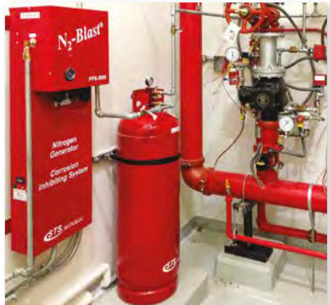
South-Tek N 2 -Blast® Nitrogen Generator fitted to a Reliable Model DDX PrePak Preaction System and Model DDX Preaction Valve.
